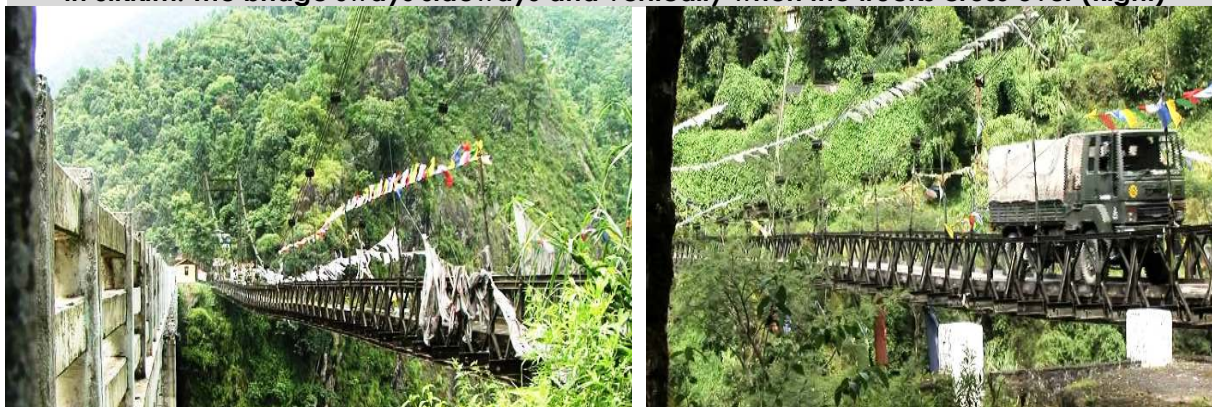
Rang-Rang bridge and Sikkim Orchids (Left). Military trucks crossing the Rang-Rang bridge in Sikkim. The bridge sways sideways and vertically when the trucks cross over (Right)
